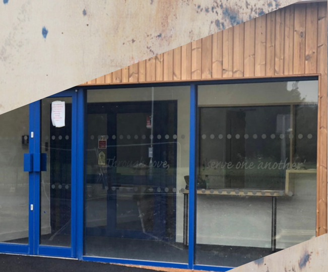
New school entrance at Bemerton St John
